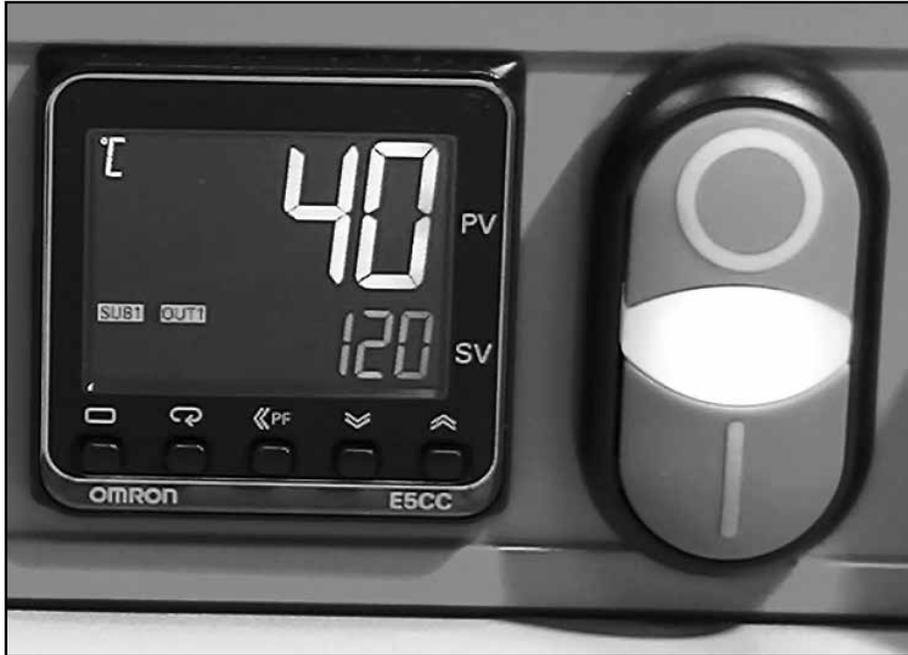
Factory preset “splice start” temperature is 40°C. A white light on start/stop switch will illuminate when control temperature is at or below setting.
